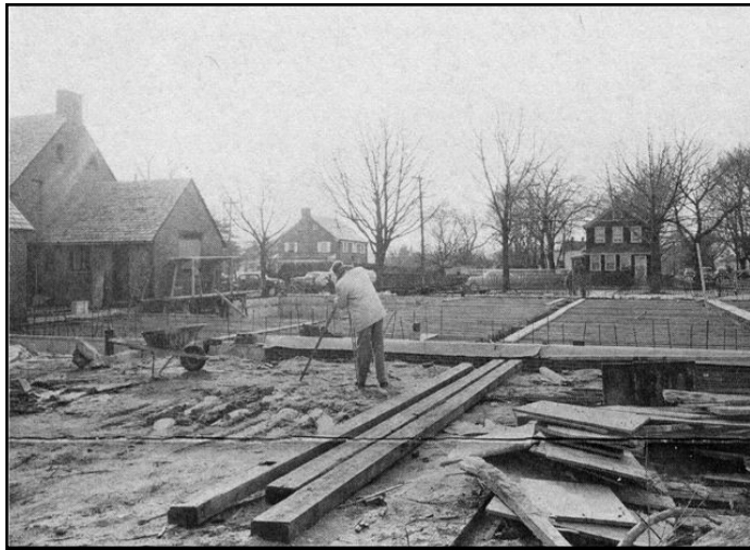
Hicksville Library Under Construction
